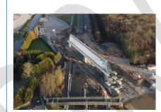
Photo of the HS2 Marston Box Bridge being installed over the M42.
