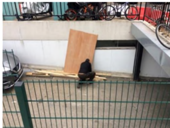
Photo of MoP cutting and collecting wood on live site access ramp.
