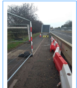
Photo of temporary access arrangements in the vicinity of roadworks.
