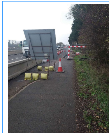
Photo of temporary access arrangements in vicinity of roadworks.
