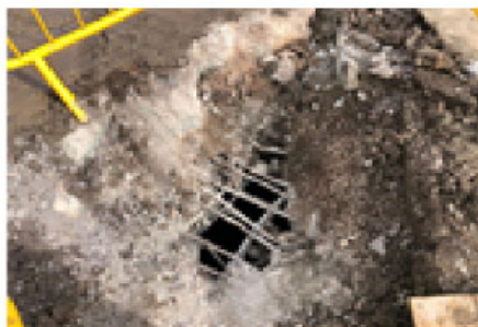
Photo of damaged Culvert soffit
