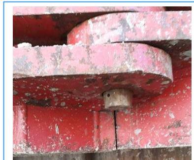
Photo of missing safety clips from a retaining pin.
