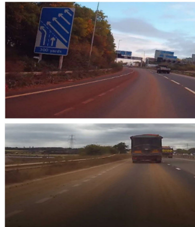
Road network adjacent site exits showing extensive covering of tracked material across lanes.
