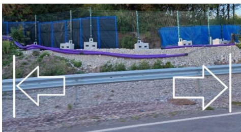
Section of cable ducting removed without approval.
