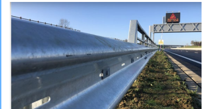
Photo of barrier set back from drainage
