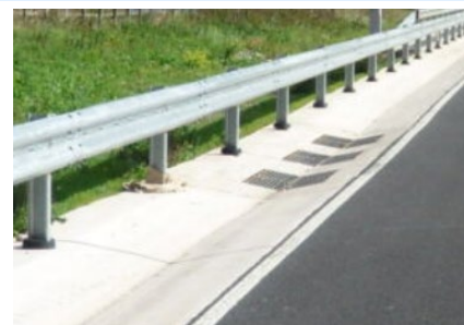
V channel installed adjacent to vehicle restraint system.
