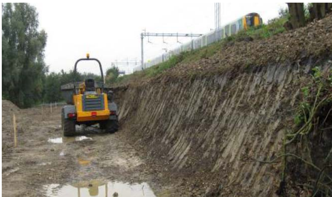
Plate 25: Bradwell Abbey toe cut contrary to (emerging) design, affecting track geometry (15 October 2013)
