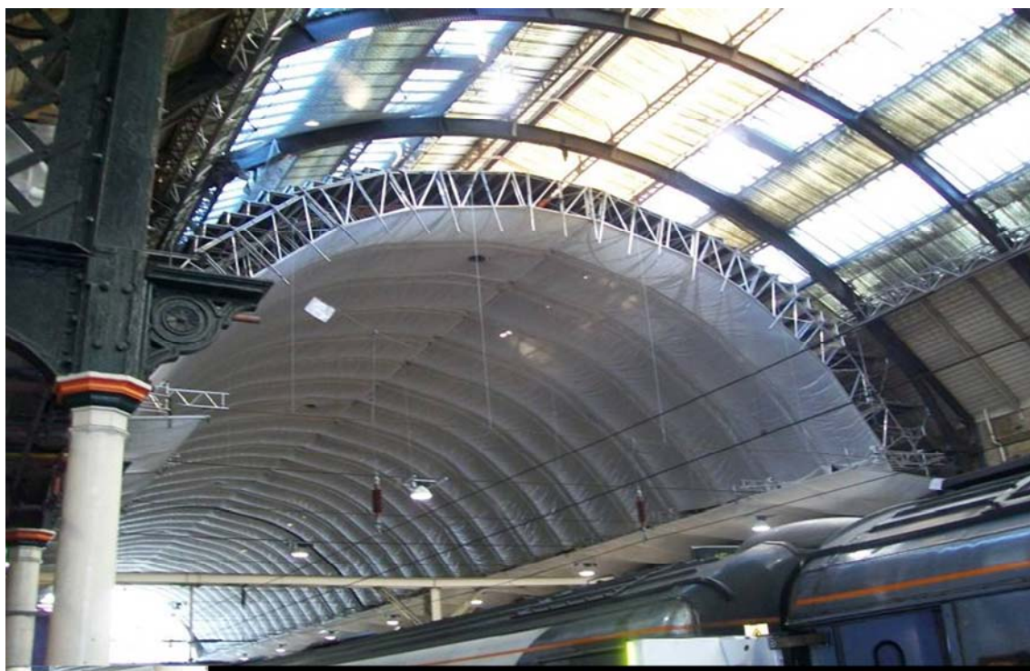
Plate 13: Operational Station with Suspended Protection Deck.
