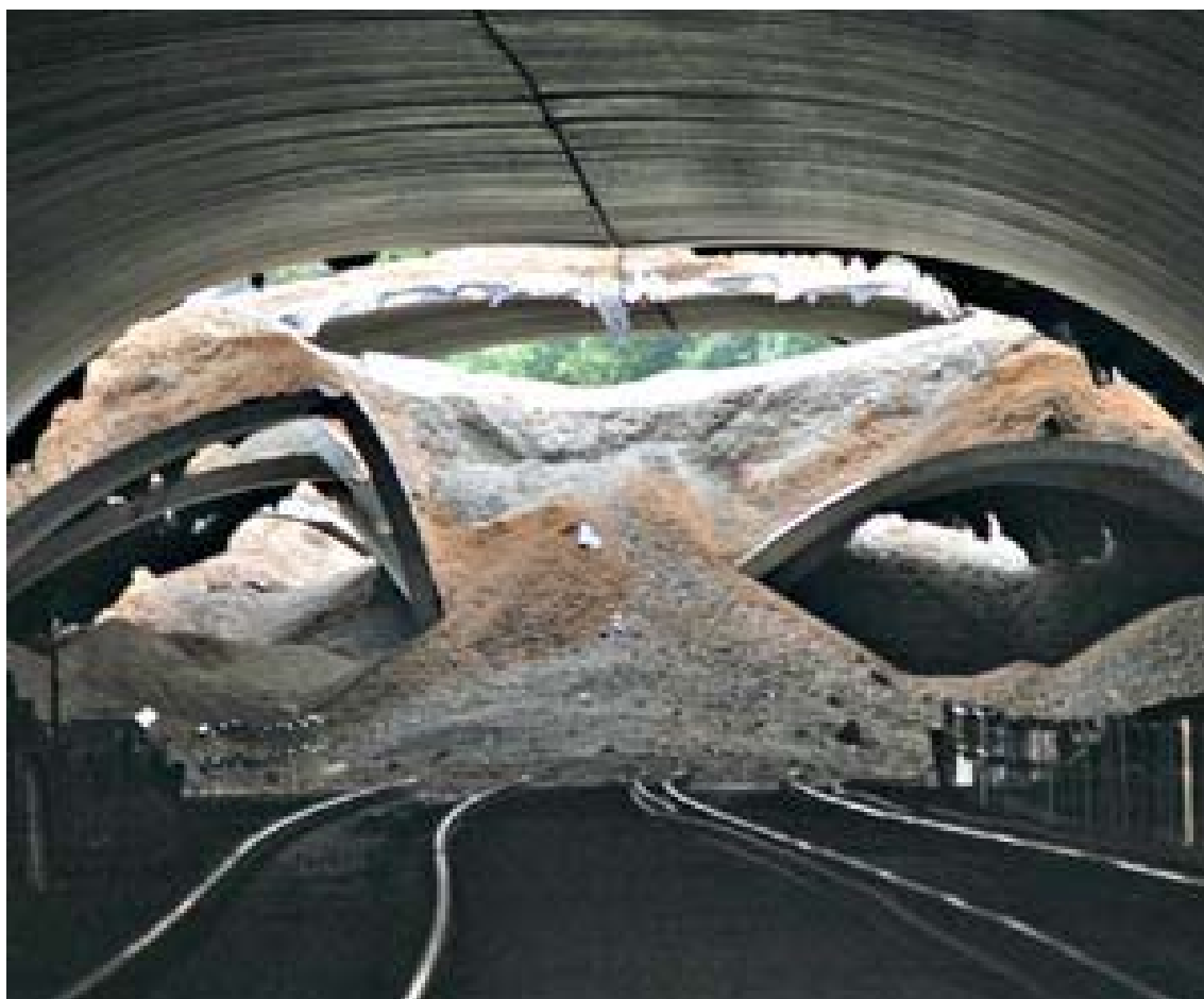
Plate 6: Collapse of Gerrards Cross Tunnel during construction.
