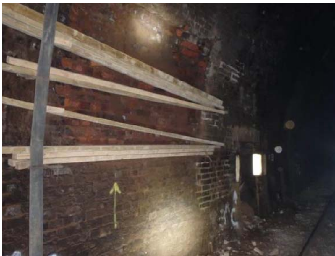
Plate 19: Temporary works in tunnel struck by train.
