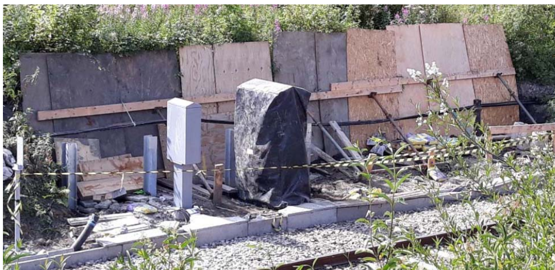
Plate 23: Breich, Scotland. Very poor Temporary Works with no design.
