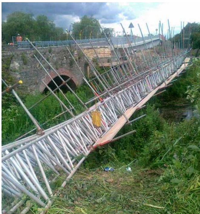
Plate 1: Collapsed Scaffold
