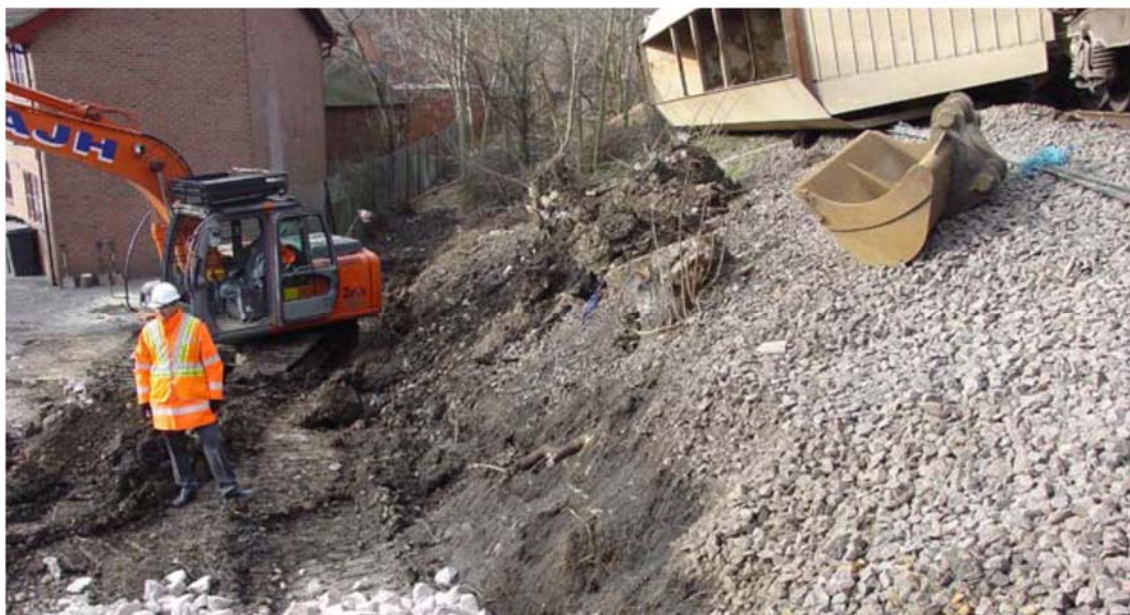
Plate 24: Temporary excavation to create works access road and site of derailed freight train at Cricklewood.
