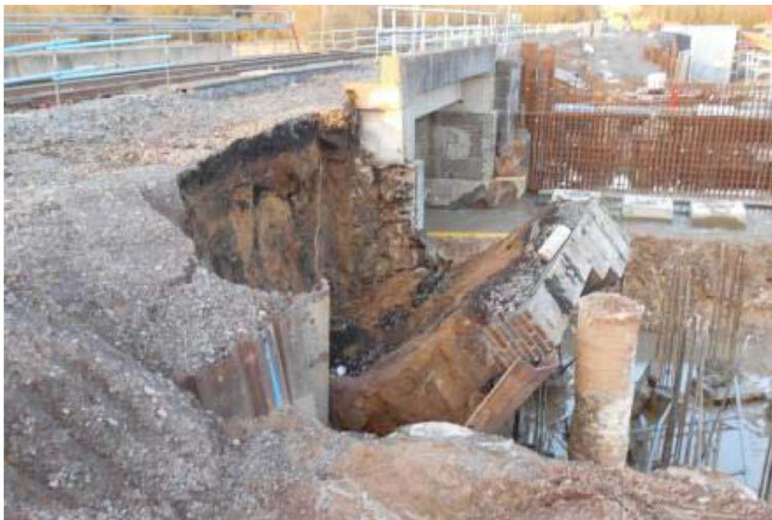
Plate 21: OXD39 Wingwall Failure due to undermining of existing structure during Temporary Works excavations.
