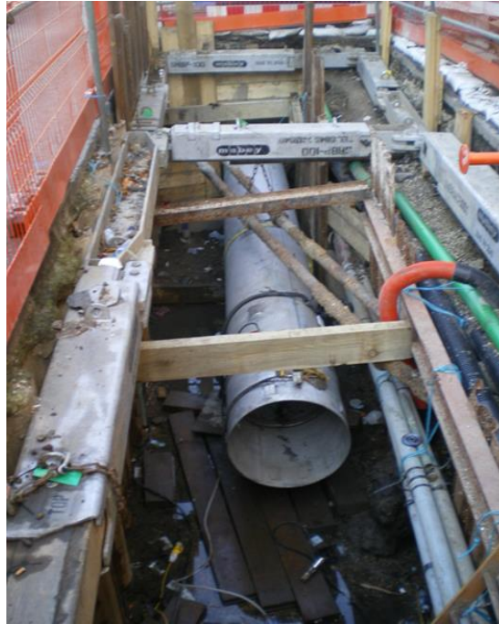
36" diam. trunk main protection works
