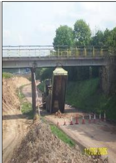
Photos (left): Result of an ADT travelling along a haul road with the Tipper equipment not correctly stowed, striking an existing footbridge, on a highways scheme in 2005.
