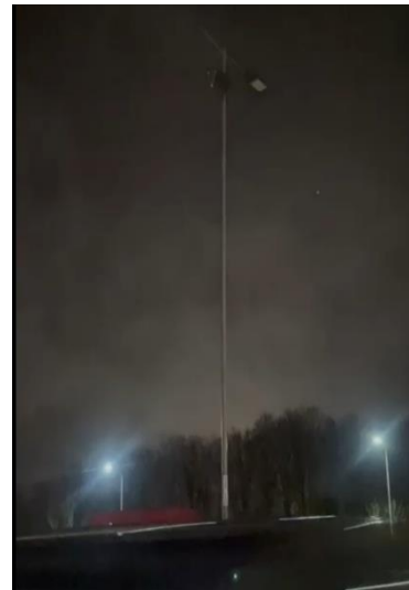
Lantern detached and hung by lanyard During Storm Henk
