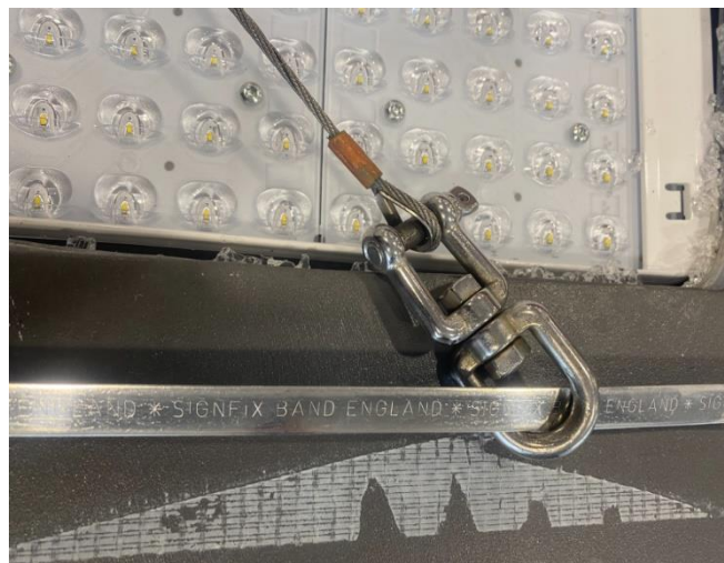
D-Shackle fixing detail
