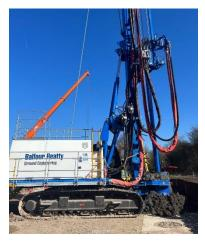
On Thursday 6 July 2023 at our AWE Aldermaston site, following the successful completion of concrete pumping on a Casagrande B300 continuous flight auger piling rig, the piling team commenced work to clean the concrete pumping system using compressed air. During this cleaning operation, a blockage was encountered.
