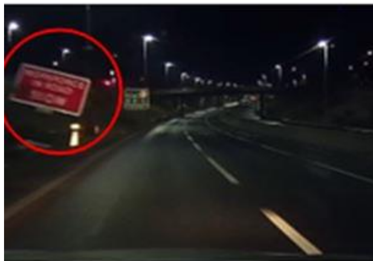
Example of incorrect sign placement
