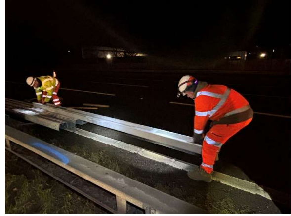
Figure A1 Installing crash barriers is a physically demanding task, requiring loads to be lifted from close to the floor. Other aspects of the task such as cutting old barriers out or securing fixings also require prolonged forward bending (pictures courtesy of Carnell Group)
