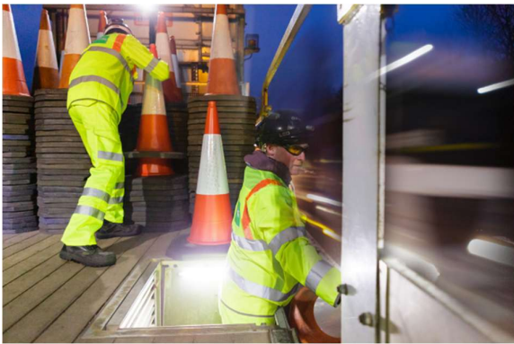
Figure A3 Team of two operatives laying traffic cones for TTM at night. (Photograph courtesy of HW Martin)
