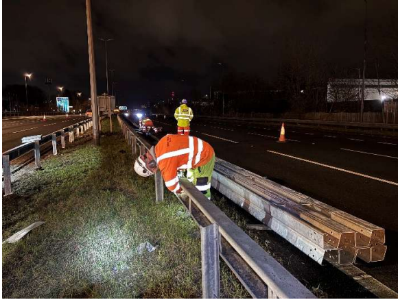
Figure A1 Installing crash barriers is a physically demanding task, requiring loads to be lifted from close to the floor. Other aspects of the task such as cutting old barriers out or securing fixings also require prolonged forward bending (pictures courtesy of Carnell Group)
