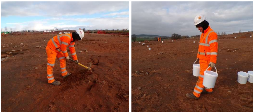
Figure A4 Using a mattock can involve working for long periods in a forward leaning position, and clay soils can require considerable force. Buckets of soil might need to be carried a long way across uneven ground
