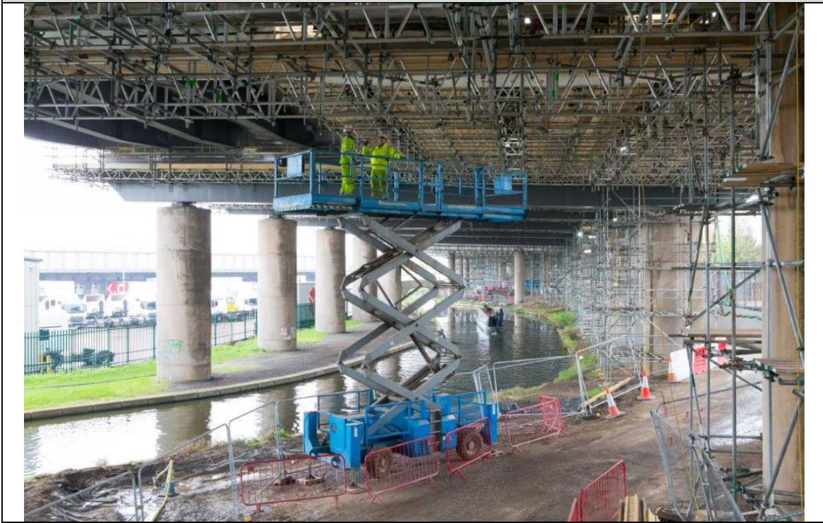
Type 3a Mobile Vertical (scissor lift) – In use at M5 Oldbury
