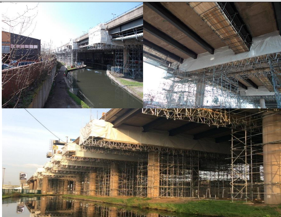
Examples of viaduct structure where MEWP's are to be used to access the soffit to affect repairs
