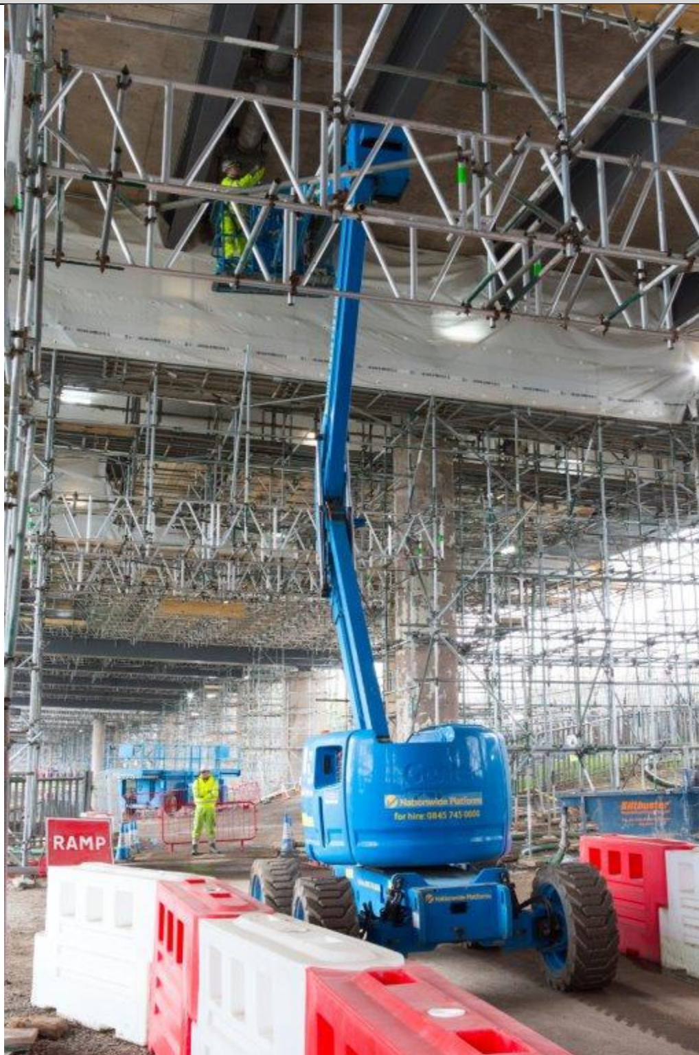
Type 3b Mobile Boom – In use at M5 Oldbury
