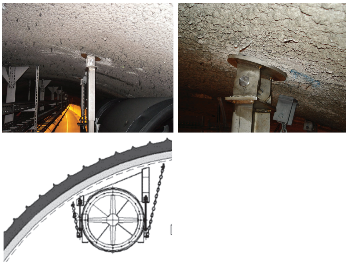
Figure 12.4 Secondary restraint chains for tunnel jet fan
