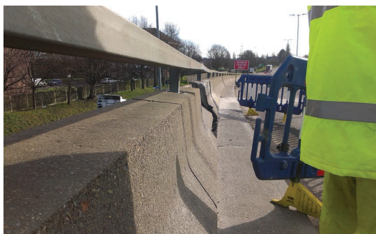
Figure 12.6 Parapet unit moved during vehicle impact
