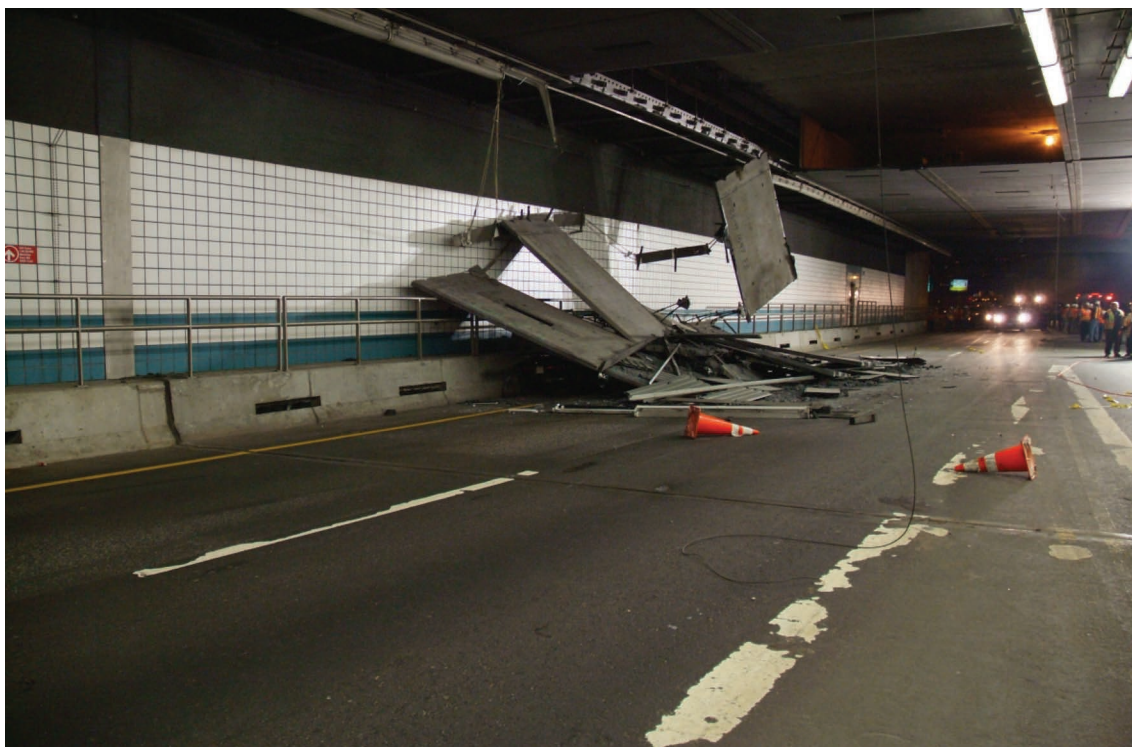
Figure 4.1 Collapse of a suspended ceiling, Boston USA (courtesy US National Transportation Safety Board)
