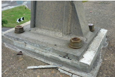
Post-installed parapet fixing
