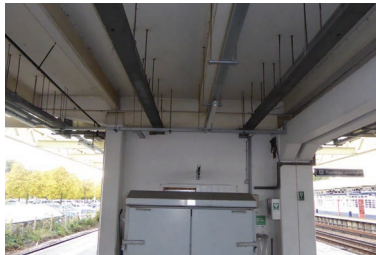
Cable trays suspended from station canopy (could be non-safety critical)
