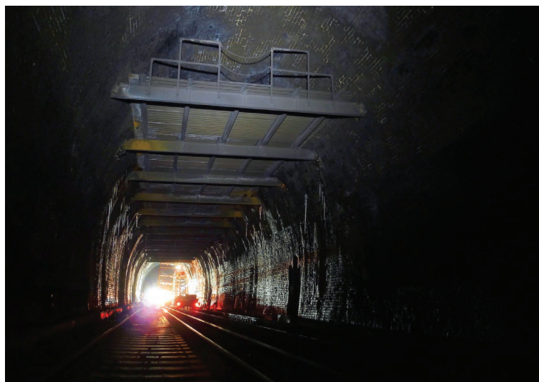
Figure 12.3 View of water catchment tray showing longitudinal beams (from RAIB, 2014)
