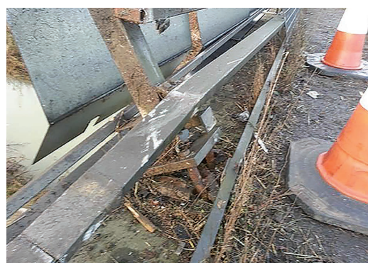
Figure A4.2 Vehicle restraint system showing post-installed fixings that had pulled out of the base
