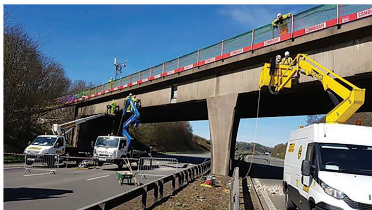
Figure 8.1 Damaged fixings to suspended fascia panels
