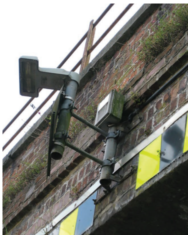
Lightweight sign, lighting and bracket fixed to bridge spandrel
