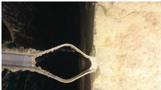
Figure 13.1 One of a series of wall ties with inadequate (zero) embedment (from Cole, 2017)
