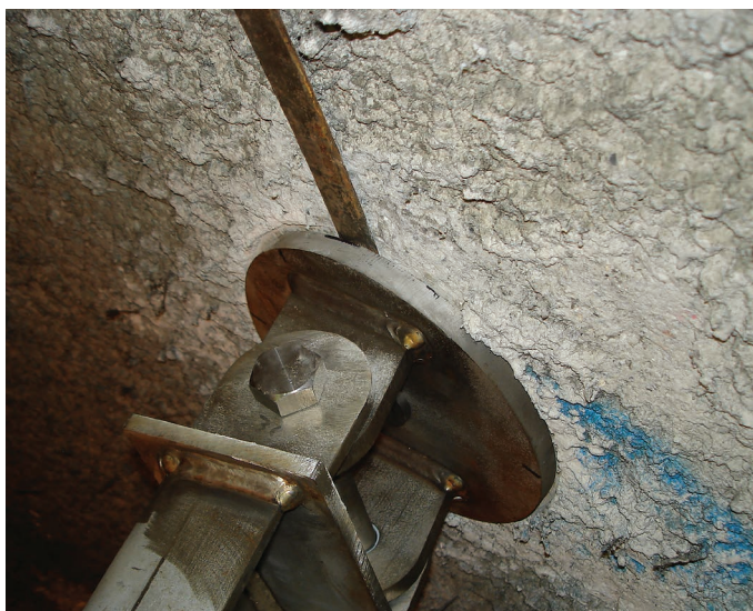
Figure 7.3 Steel ruler inserted into gap between anchor plate and concrete substrate of tunnel lining
