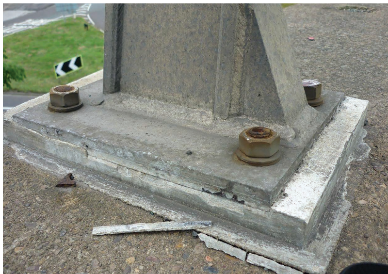
Figure 5.2 Post-installed parapet fixing
