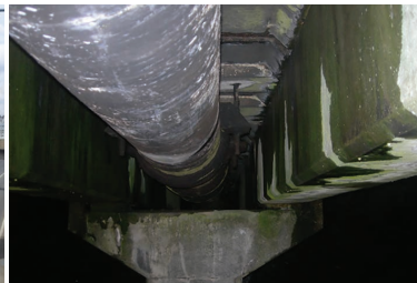
Utility suspended from bridge deck
