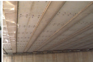
Infill panels on bridge soffit
