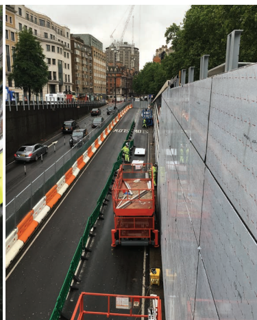
Cladding system in underpass
