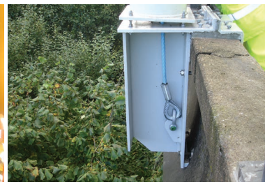
Gantry attached to bridge parapet
