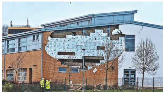
Figure 13.2 Collapse of part of the outer skin of a cavity wall at a school during high winds, with nine tonnes of masonry falling into the playground (from Cole, 2017)
