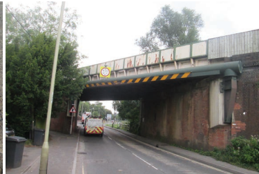
Bridge collision protection beam
