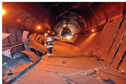
Figure 12.5 Progressive collapse of a 140 m length of ceiling panels in Sasago Tunnel
