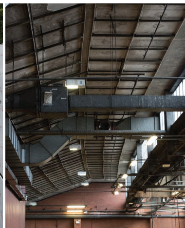
Ventilation system in bus depot
