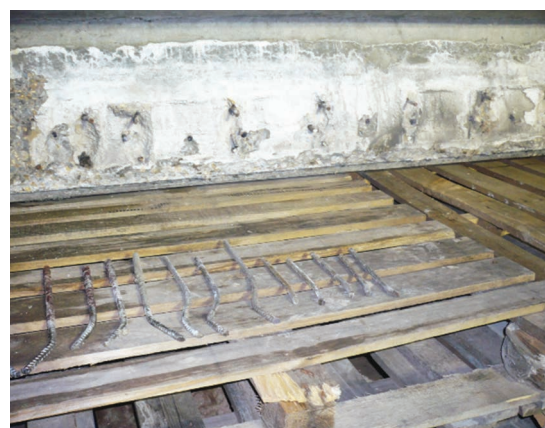
Figure 12.7 Loose resin anchors laid alongside parapet unit (courtesy Southampton City Council)
