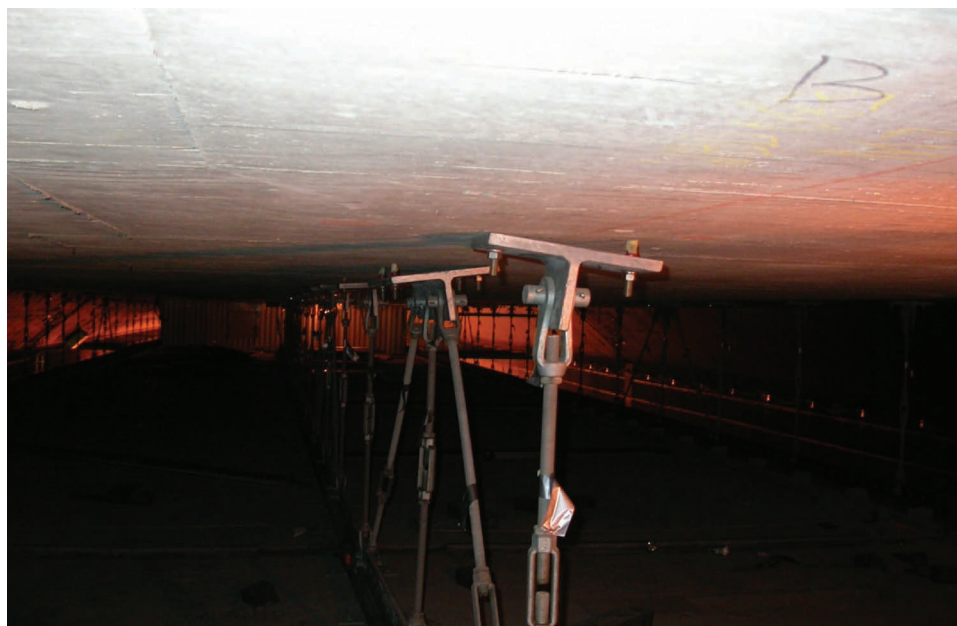
Figure 7.2 Deformation of fixings, Boston, USA (courtesy US National Transportation Safety Board)
