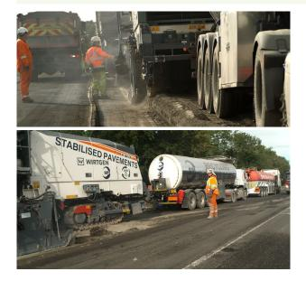
Work began on site on September 25th with pre-planing carried out at 60mm in order to accommodate the new surface material depth of 40mm as well as the potential bulking from the recycling process. The Wirtgen 380CRi was deployed and mixed pre-spread blended PFA/Cement and introduced foamed bitumen within the mixing chamber to create the recycled foundation.
