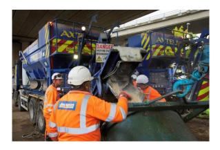
A team from Jackson, concrete supplier DB Group and Axtell scaled up the use of Cemfree using a volumetric mixer or mobile concrete batching plant.
