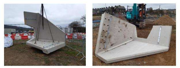
Precast headwall sections were procured for installation into the works. The units were supplied with lifting points installed during manufacture. Although the units were successfully unloaded on delivery, when lifting at the later stage a unit had only just cleared the ground when it rolled over and fell onto the wing wall. Exclusion zones were in place, no injuries and no damage to plant.
