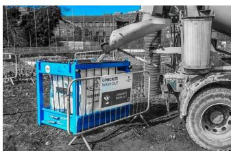
This system allows a person to wash the wagon chute into a 'BlueRinse Nappy Sack' filter; solids are contained, and the water passes through the sack, which has an alkali reducing agent impregnated into the lining. No power source is required, and a hose can be attached to allow the filtered water to flow to a discharge point.
