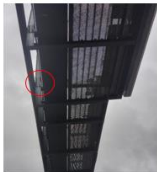
Traffic sign support on portal gantry
