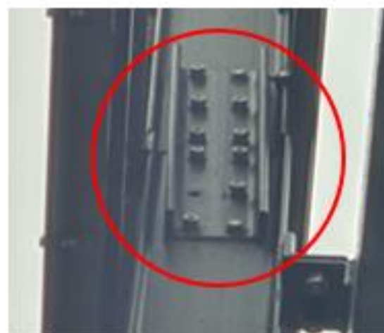
Missing/loose bolt, nut and lock nuts
