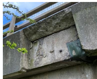
Damaged Parapet Coping
