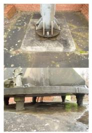
CCTV similar installation CCTV Holding down arrangement The holding down arrangement consisted of ungrouted bolts and with the base of the mast set on levelling nuts.
