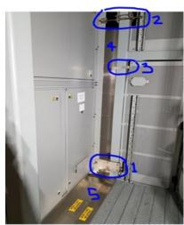
The picture above shows two friction grip brackets (1 and 2), which hold an MS4 in place on a gantry leg. Concerns were raised regarding the design of this:
