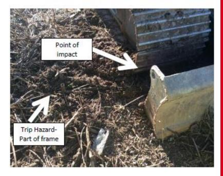
The injured person (IP) was doing pre-use checks on the excavator at the start of work and tripped on a part of a temporary sign frame protruding from the ground.
