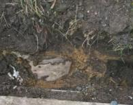
During the installation of a Distribution Network Operator Ducting, a 550mm deep channel needed to be excavated. To enable these works trial holes were dug using a RED permit. The services were identified and appropriately and clearly marked on the ground by the team.
