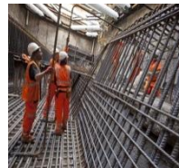
Working on Rebar
