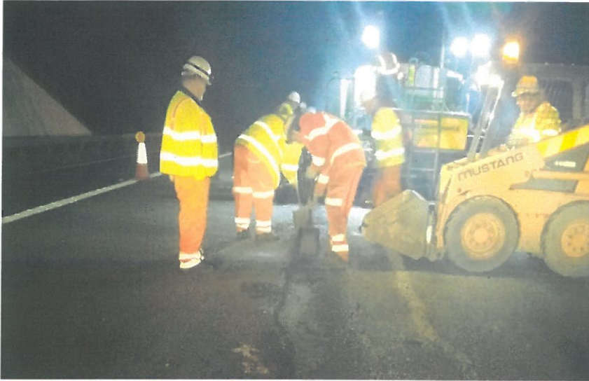
Figure 5 - Team install pre coated chippings
