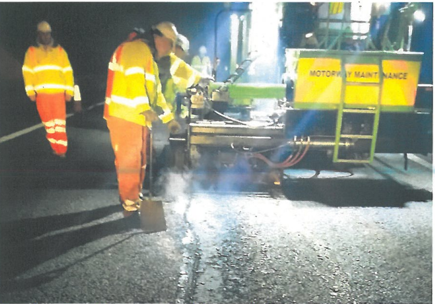
Figure 4 - equipment has passed over joint re-worked
