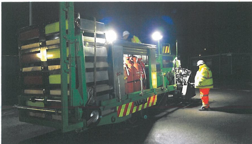
Figure 1 - Equipment off loaded on site
