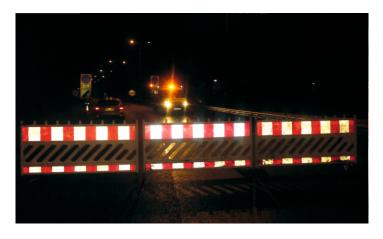
The Intellicone Safelane perimeter incursion system was innovatively used on the A180 by Aone Plus Area 12. The system which consisted of 1 full closure point, 1 checkpoint with CCTV and panic alarm and 1 contractor alarm was deployed overnight as a pre-works scheme, to allow safe implementation of the daytime network TM, site materials and plant.
