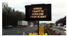
The pVMS is positioned in advance of the works exit. Works traffic exiting the site pass sensors mounted on a pair of Alert Towers (one each side of the works lane). This triggers the pVMS located within the central reserve 200 yards beforehand and flashes up a message "Works Traffic Merging From Right", warning road users that a vehicle is exiting the works to re-join the carriageway.
