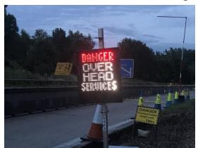
definition quattro variable message signs that activate when construction plant and vehicles approach an overhead service and or hazard.
