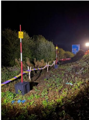
To aid identification throughout the life of the temporary cable, in addition to maintaining clear access to the cable, the installation of hazard markers is recommended. The hazard markers should be placed at the start and finish of the safety critical cable and at regular points along the route to provide an enhanced visual identifier.
