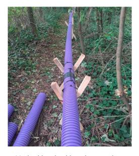
Wherever possible, temporary safety critical cables should not be routed within 2m of the vehicle restraint barrier or edge of carriageway (e.g., to avoid damage through vegetation clearance or placed within VRS deflection zone). The Design Risk Assessment and planning activities must consider routing the cable away from the carriageway, along the rear boundary if access for installation and maintenance is possible.
