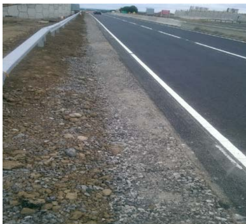
A1 Leeming to Temporary Narrow Lane Running A1 Barton example of verge hardening and temporary raised rib line
