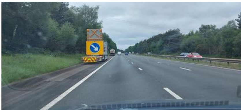
Figure 1 Single Vehicle moving works on a hard shoulder typically at risk of collision from traffic inadvertently leaving the carriageway 'drifting'
