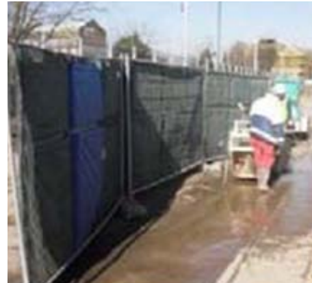
Floor sawing behind acoustic screen
