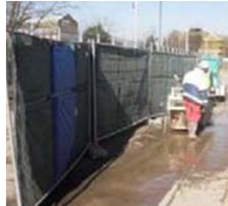
Floor sawing behind acoustic screen
