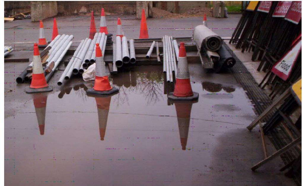
**This photo shows a storage area with a pool of rain water being allowed to develop. Not only is it a hazard in its own right, think about freezing temperatures!**
