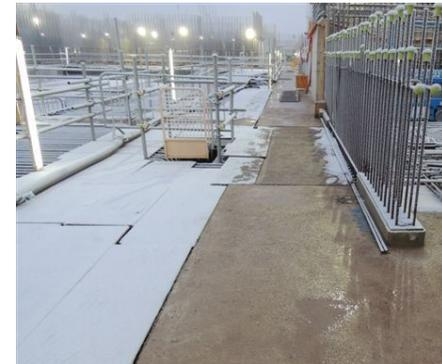
**An example of use of a sprayable de-icer solution in action**
