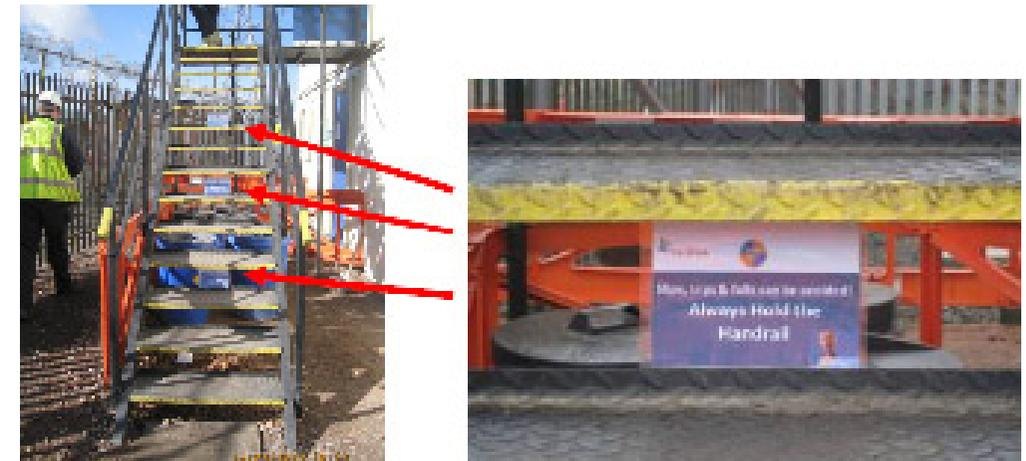
Example of a sign displayed under the steps or on landings to remind users of the requirement of holding the handrail
