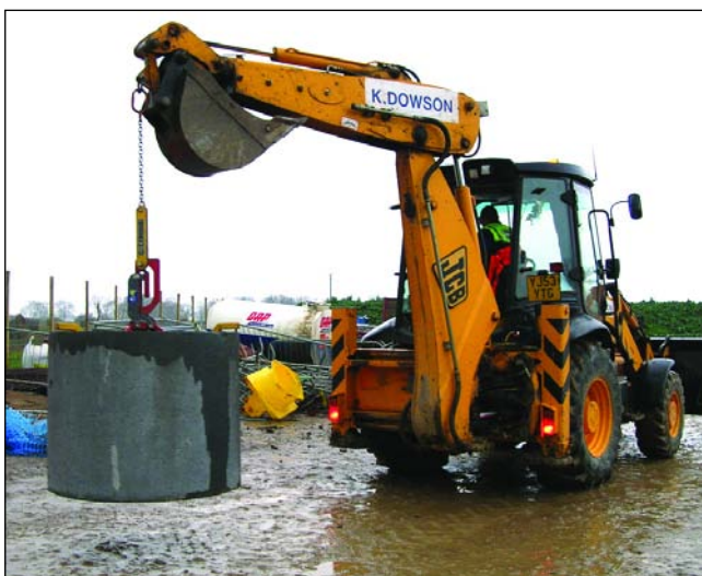
Figure 1 Lifting safely thanks to the three-pronged device
