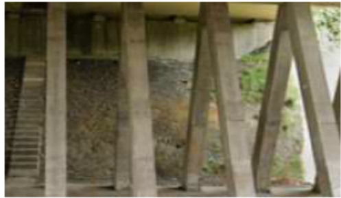
Photo of a bridge revetment without surface stabilization treatment
