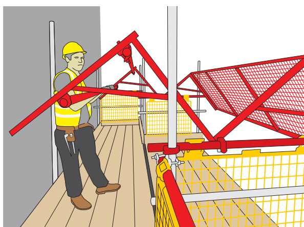
Figure 42: Example of a loading bay gate to maintain collective fall protection for the scaffold users when the loading bay gate is open.
