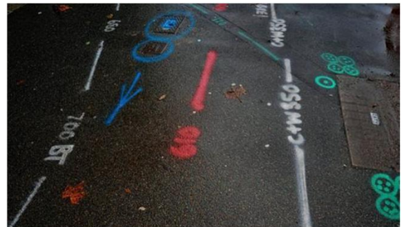
Surface marking of surveyed utilities
