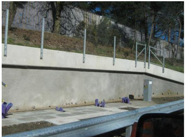
Replacement for the bored Piles
