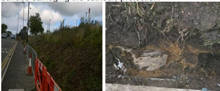
During the installation of a Distribution Network Operator Ducting, a 550mm deep channel needed to be excavated. To enable these works trial holes were dug using a RED permit. The services were identified and appropriately and clearly marked on the ground by the team.
